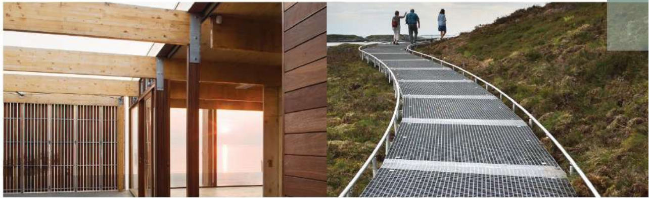
Hardwood timber - plantation - grown and recycled timber treated for protection from insects and decay - Red Gum, Jarrah and Tallowood are most durable and suitable for structure is the water. Photo: John Gollings
