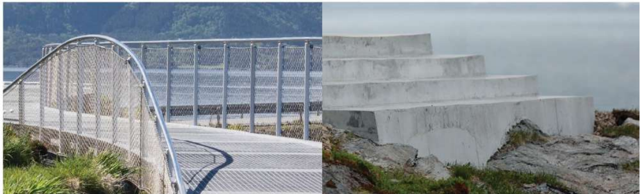
Steel - structural grade and hot dip galvanised as per AS/NZ 4680 for superior performance and powder coated for corrosive protection. Photo: Jarle Waehler
