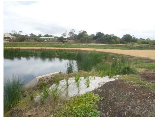
Recently constructed and planted wetland at the end of Goodall Street
